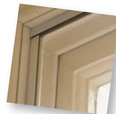
Sash windows are notorious for letting in cold air. You can get clear, light-weight acrylic panels to fit over the glazed frames, but these don't cover the many gaps on the sides, top and bottom that make sash frames particularly draughty.
