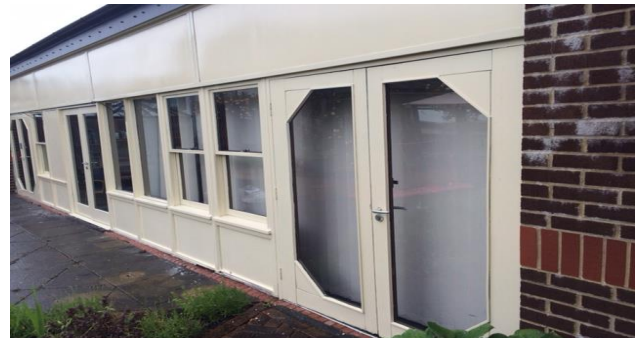
Sobell House Hospice after refurbishment.
