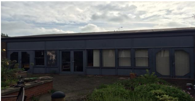
Sobell House Hospice before refurbishment.
